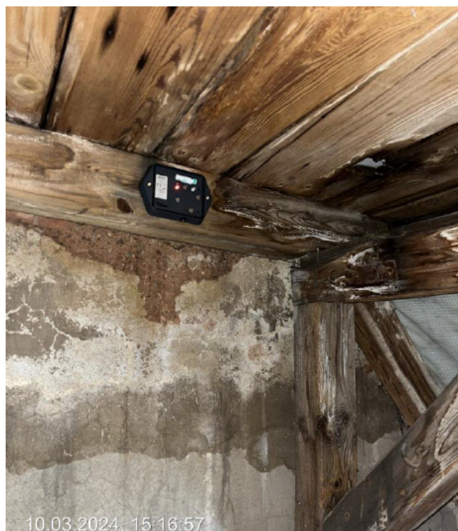
Figure 4. Positioned moisture measurement sensor at the support point in Werday
