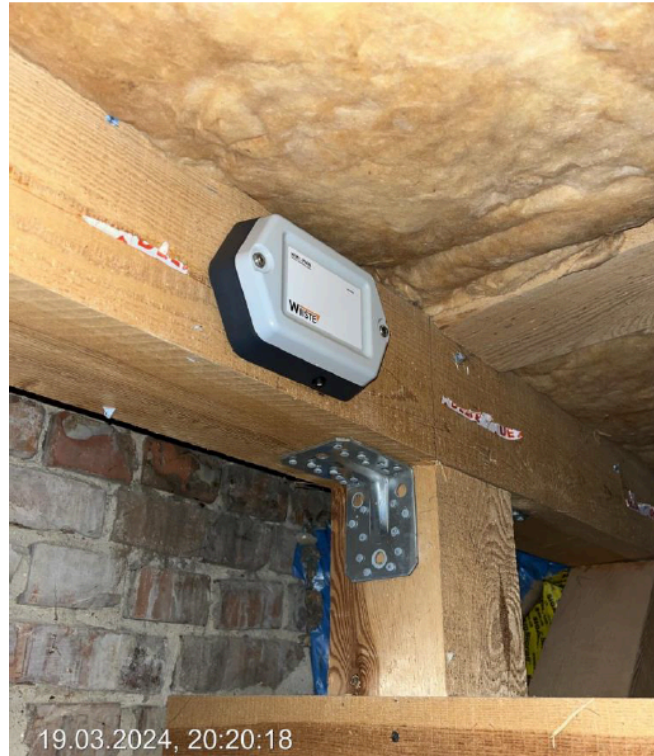
Figure 3. Positioned moisture measurement sensor at the support point in Pankow
